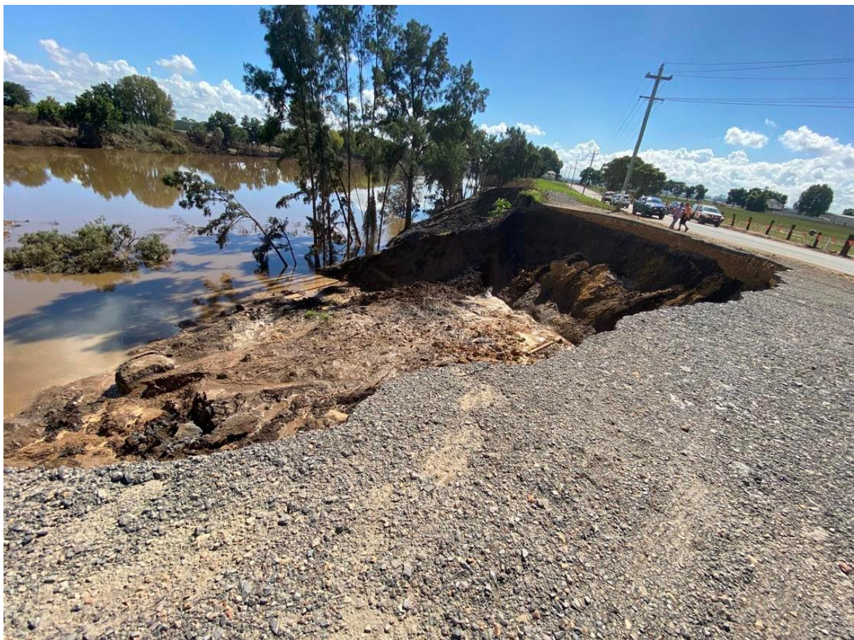
Figure 5 - Riverbank collapse threatens road infrastructure, Freemans Reach Road Hawkesbury City Council
