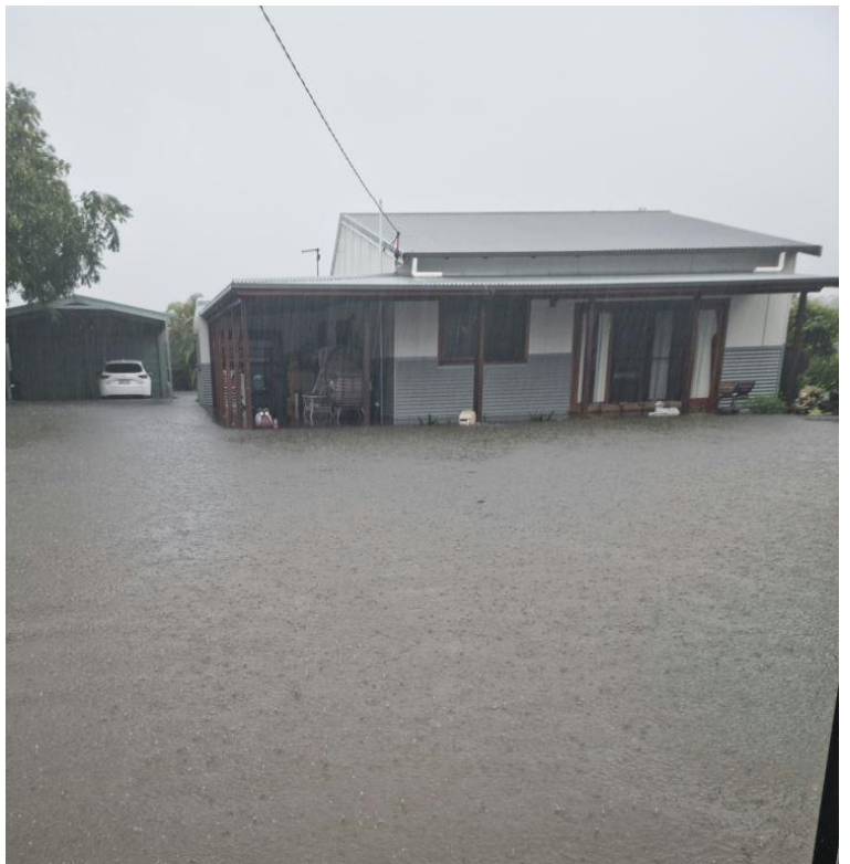
1b. House 125 Yamba Rd Stormwater 2 March 2022
