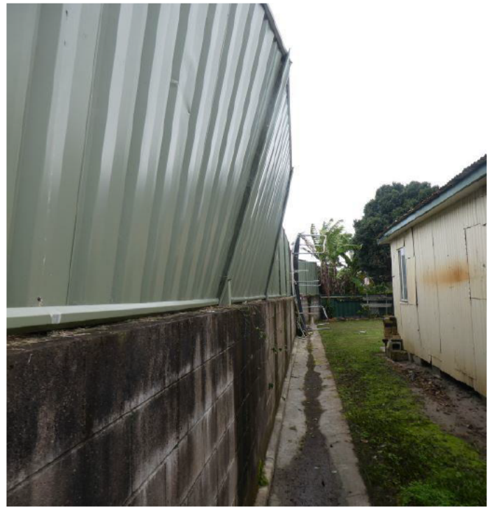
3b. 135 Yamba Rd fence broken from pressure of storm water
