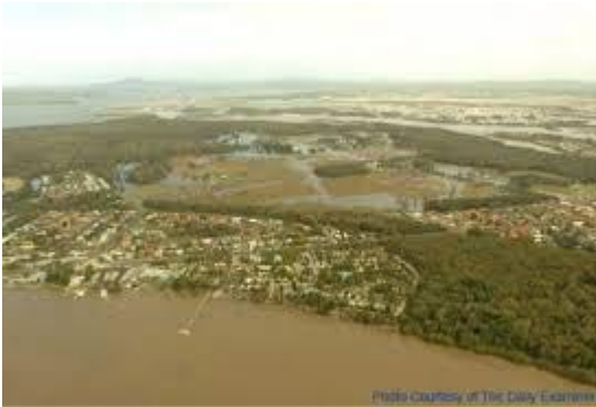
Prior to fill - West Yamba Floodplain
