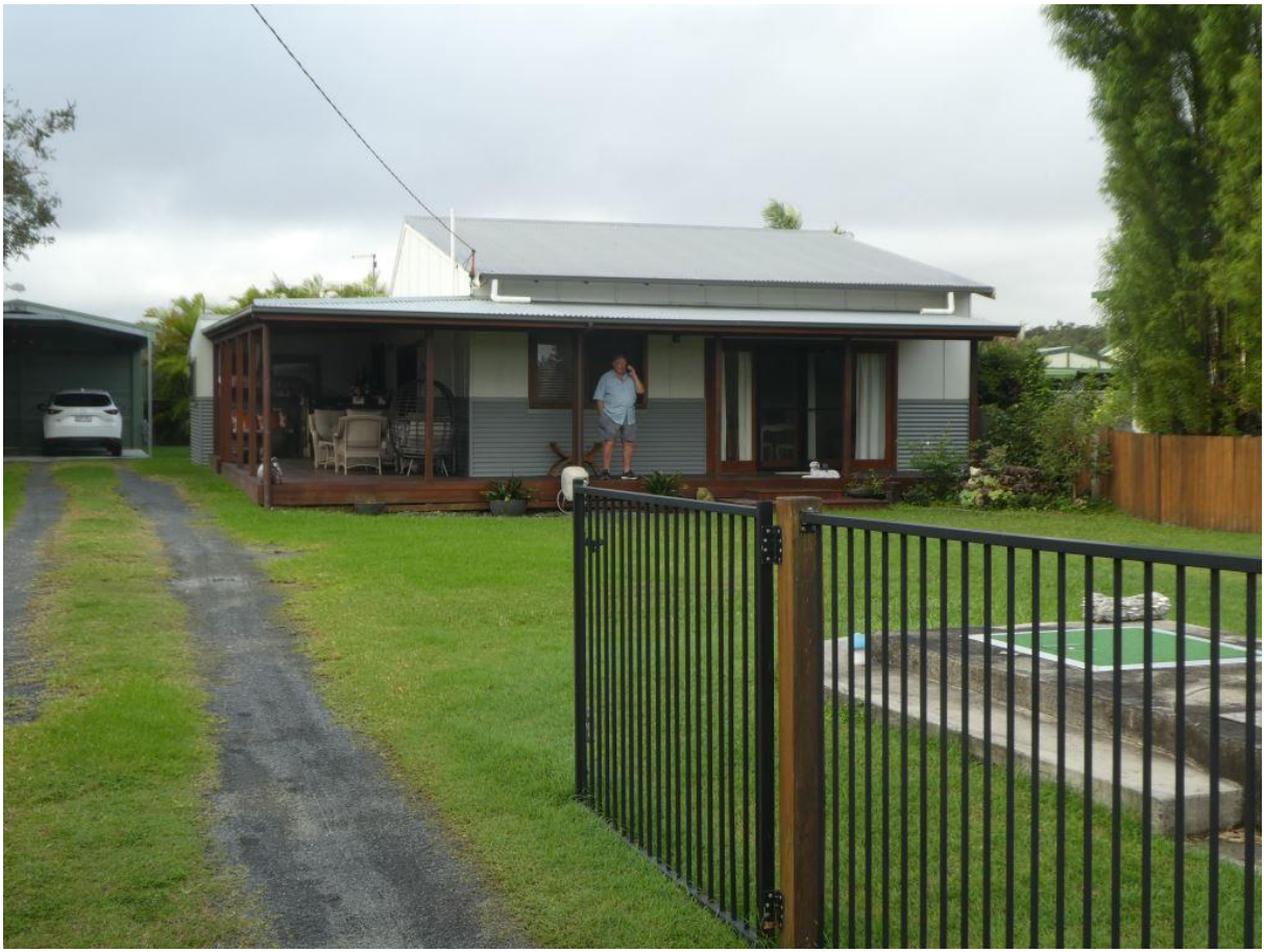
1c. House 125 Yamba Rd 16 May 2022
