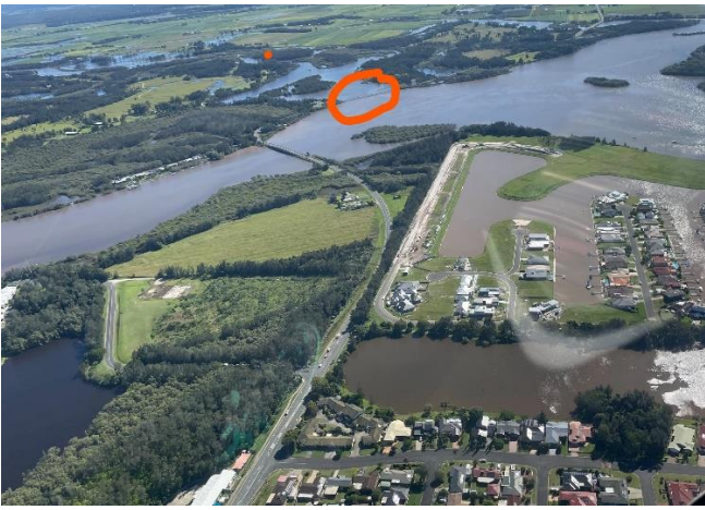
Yamba One Road OUT – over Shallow Channel Causeway
