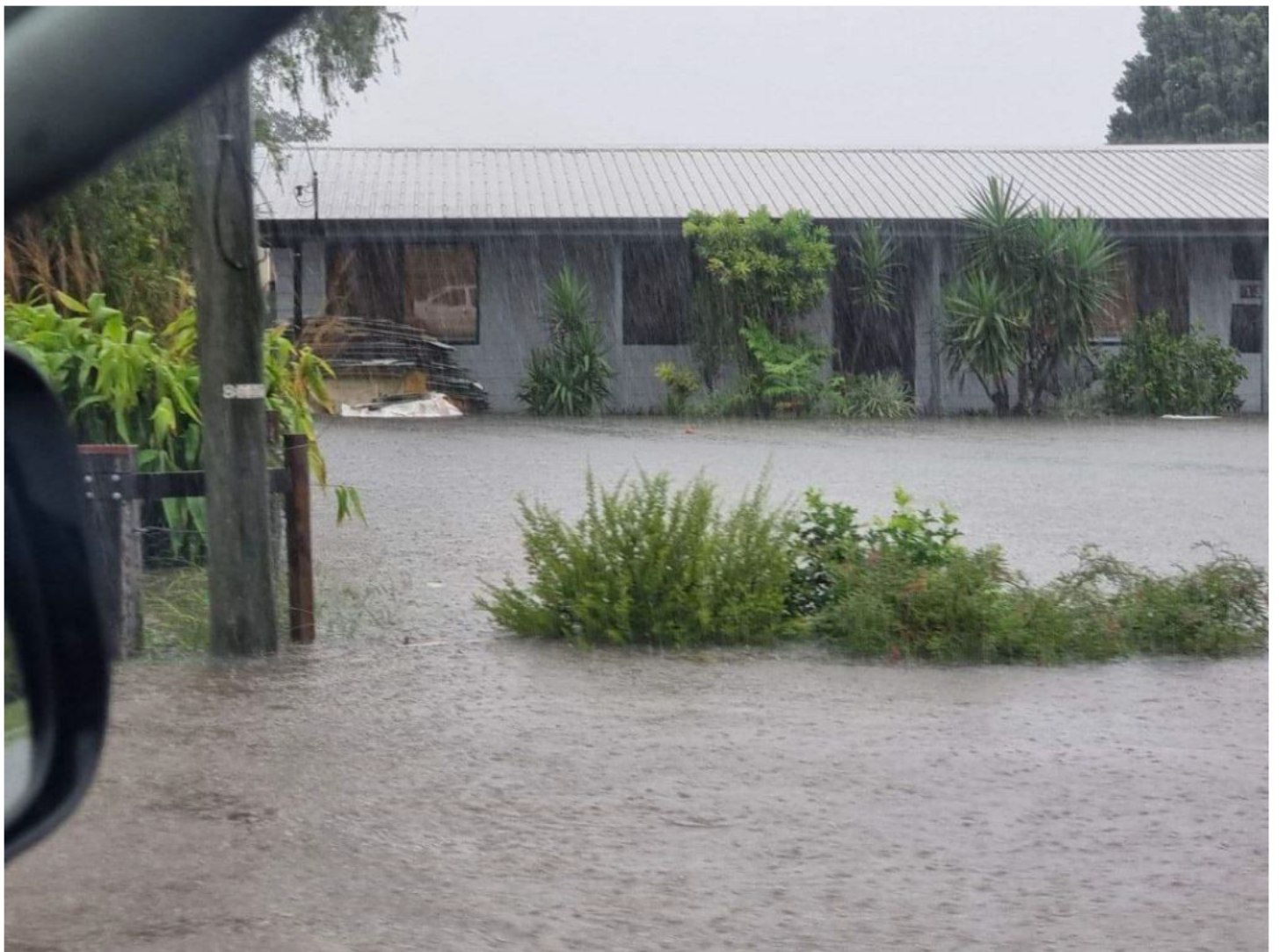
3c. 135 Yamba Rd Storm Water 30cm high through home
