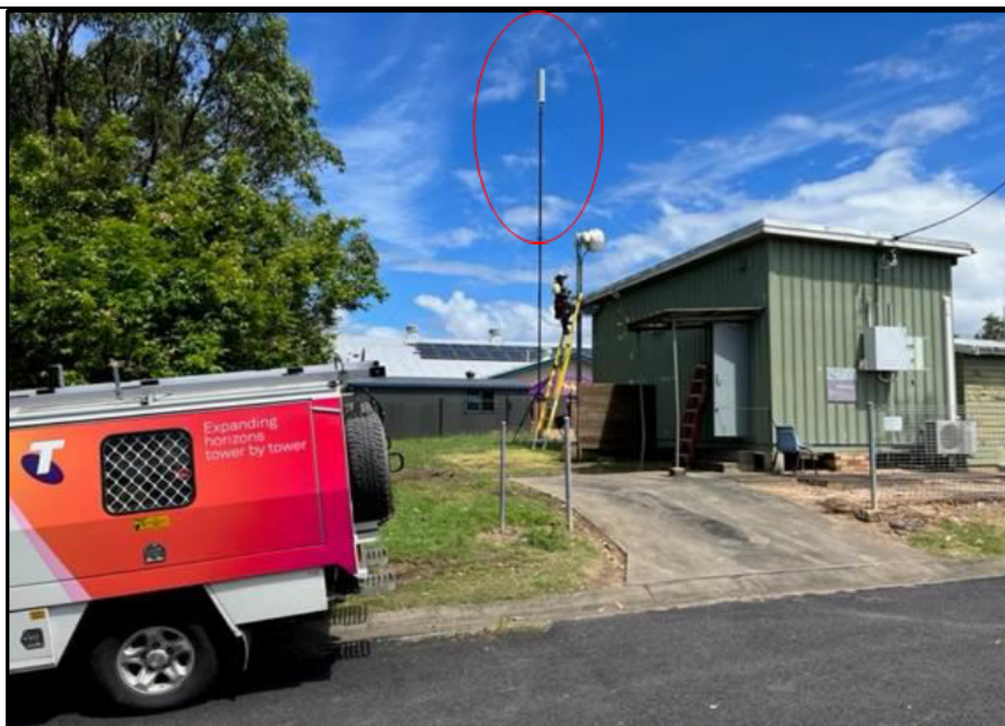
Figure 8: View of the Woodburn Exchange with the antenna of the COW visible behind the exchange building (red circle).
