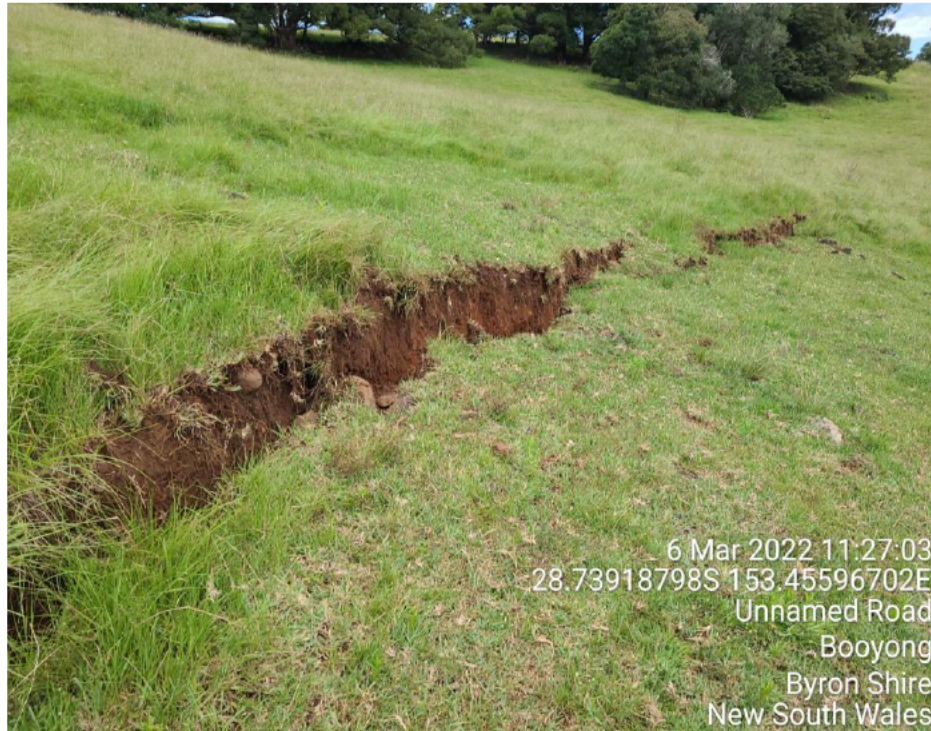
Figure 1: Land slip in Booyong NSW that damaged an optic fibre cable.
