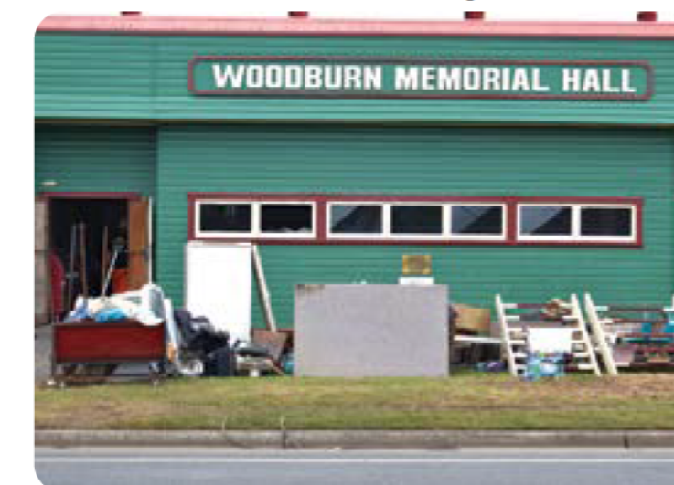
Flood damage at Woodburn Hall
