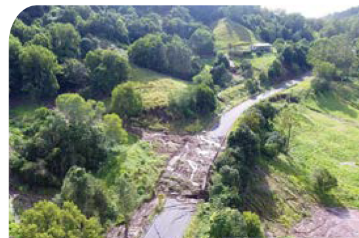
Naughtons Gap Road landslip
