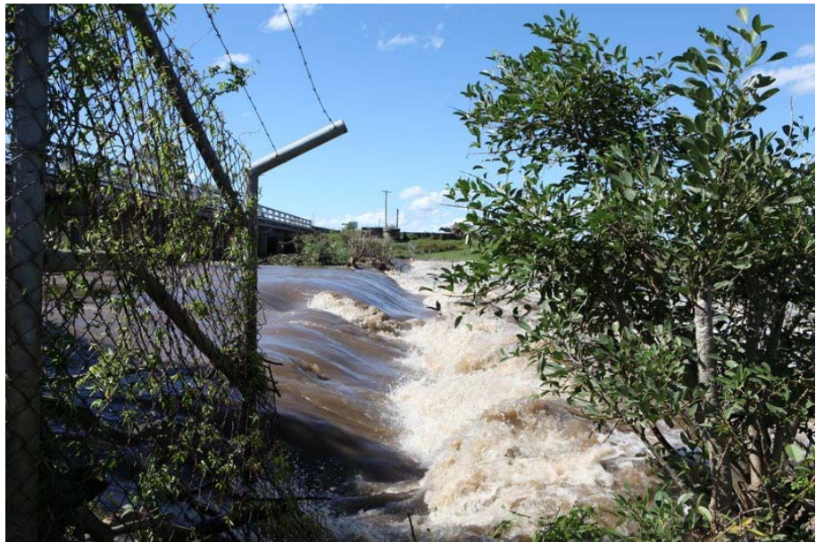
Fig 10 Concrete weir obstructing flow
