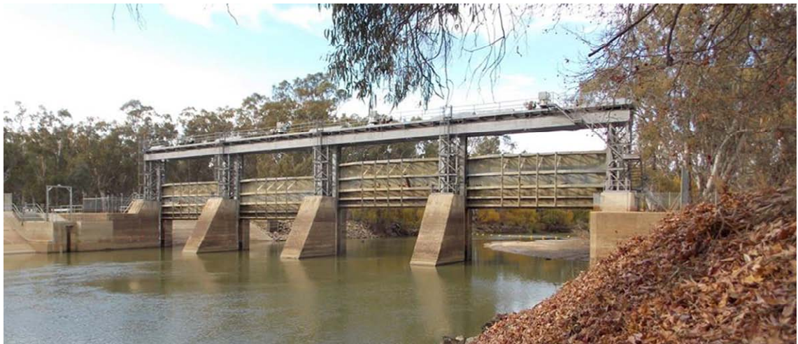
Fig 15 Stevens Vertical Lift Bulkhead Weir
