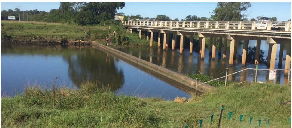
Fig 16 Tuckombil Canal Fixed Concrete Block Weir
