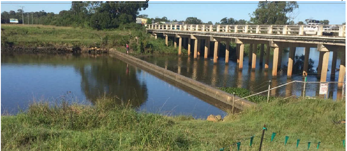
Fig 7 Present Fixed Height Weir 2019
