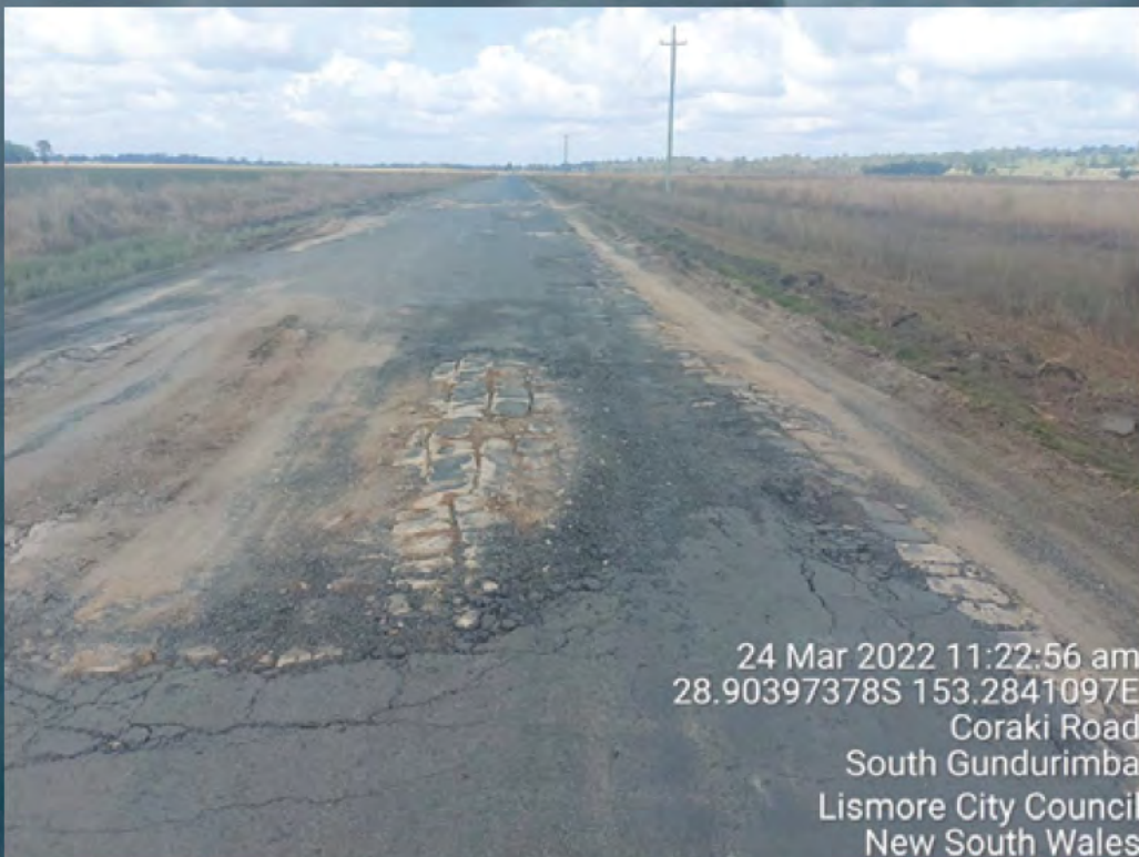
Coraki Road: Pavement damage caused by haulage of flood waste
