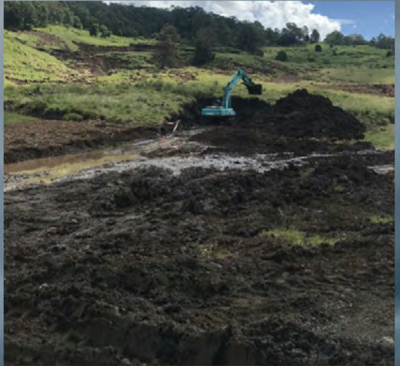
24t excavator clearing landslide over Bice Rd, Leycester
