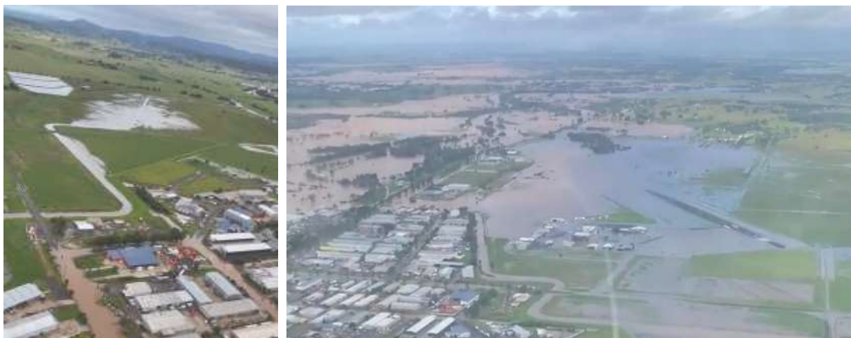
Figure 5: Photos by Rotorwing Helicopter Services 8 showing two views of these engineering works: (left, 10am 31-3-22) looking northwest across the completed earthworks (top centre), with the sewerage works top left, Leycester Creek top right, and zig-zag drain bottom left; (right 30-3-22) looking south across the partially-flooded airport towards the Bruxner Highway, showing the zig-zag drain filled to capacity with nowhere to flow.
