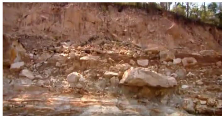
Plate 3: Erosion in Paradise Creek, Lockyer Valley, January 2011 (Lockyer Valley Regional Council)
