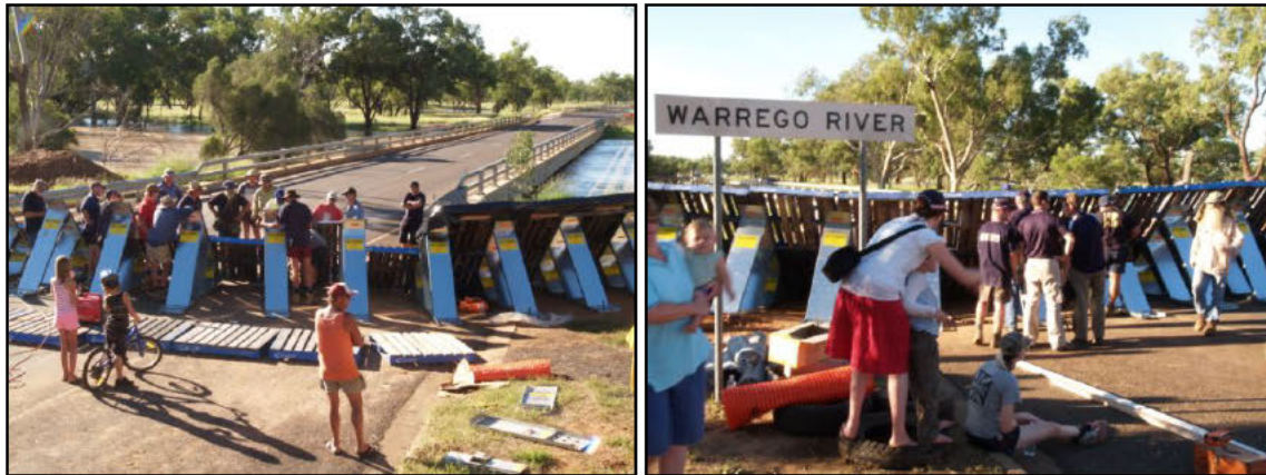
Figure 5.13. Some people in the community who helped during the construction of temporary levee during the 2008 flood in Charleville (Photo source: Chester Wilson)
