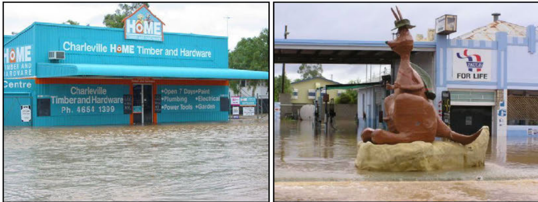
Figure 5.2. Business premises flooded in Charleville (Photo source: Charleville Home Hardware and Chester Wilson)
