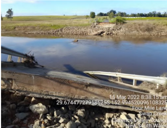
Wilcox Bridge, Four Mile Lane
