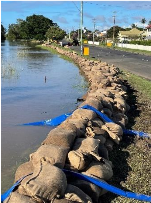
Sandbagging of levee
