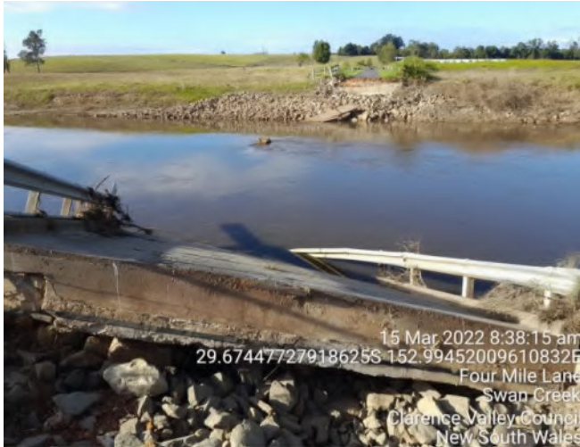
Wilcox Bridge, Four Mile Lane
