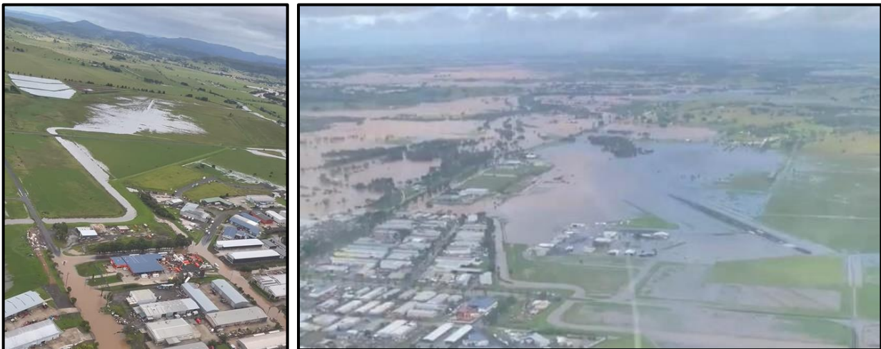
Figure 2. Photos from Rotorwing Helicopter Services 4 showing two images of these engineering works: ( left , 10am 31-3-22) looking northwest across the completed improvement (top centre), with the sewerage works top left, Leycester Creek top right, and zig-zag drain bottom left; ( right 30-3-22) looking south across the partially-flooded airport towards the Bruxner Highway, showing the zig-zag drain filled to capacity with nowhere to flow.
