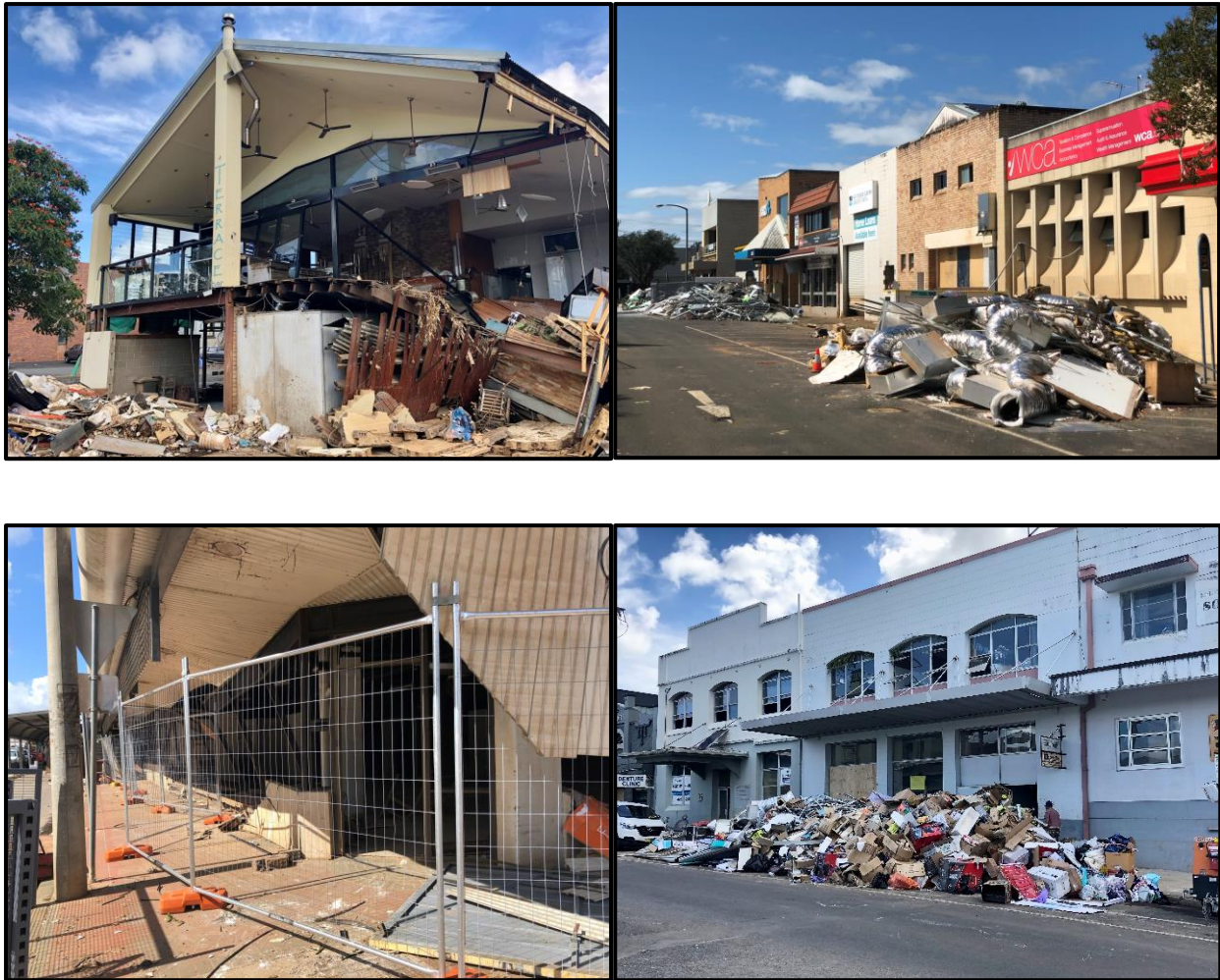
Figure 12. Businesses in Lismore’s CBD, devastated by flooding, including loss of stock, equipment, fittings and major structural damage. Photos: Barbara Rugendyke
