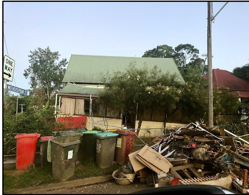
Figure 13. Dwellings sustained structural damage. Photo: Barbara Rugendyke.
