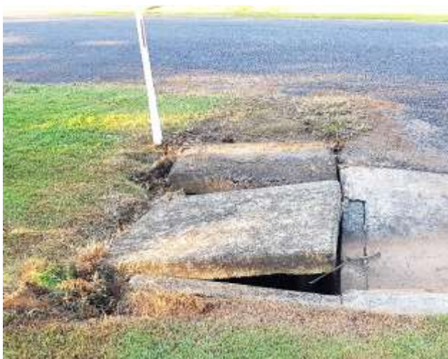
Debris line on white fence opposite showing depth of water at peak of flood..... and drain cover after flood
