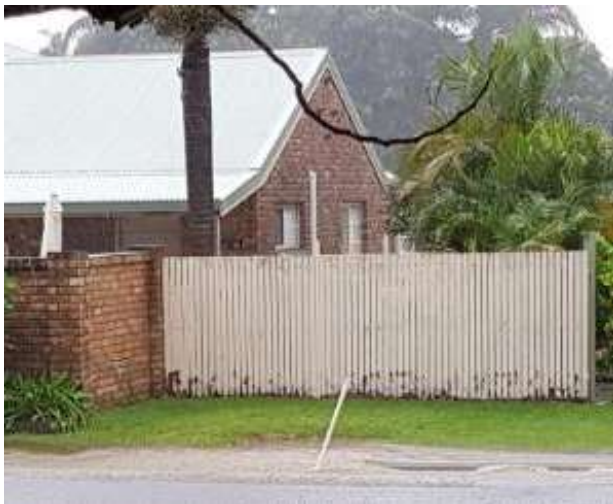
Debris line on white fence opposite showing depth of water at peak of flood..... and drain cover after flood
