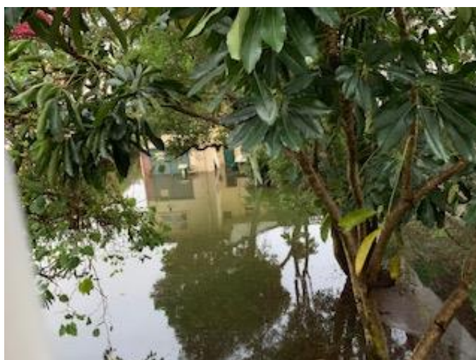
Image 5: View from balcony of unit looking to the end of [redacted] after the water had receded approx. 25cm as per water mark on wall.
