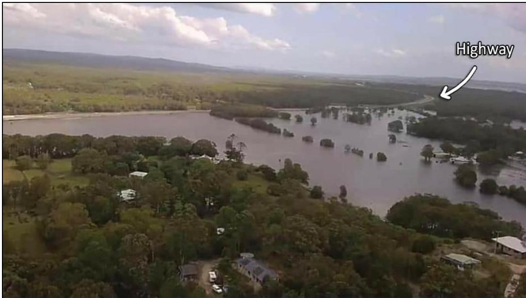
Figure 2: Aerial image of highway acting as dam
