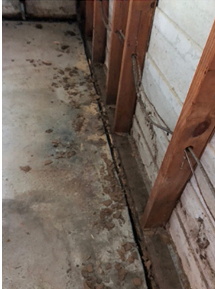
Fig 88/9 studio walls, cavity mud , lining and insulation removed, Fig 90 muddled sliding door
