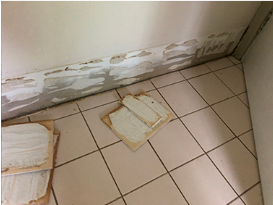
Fig 26/7 . Bathroom: tiles falling off .
