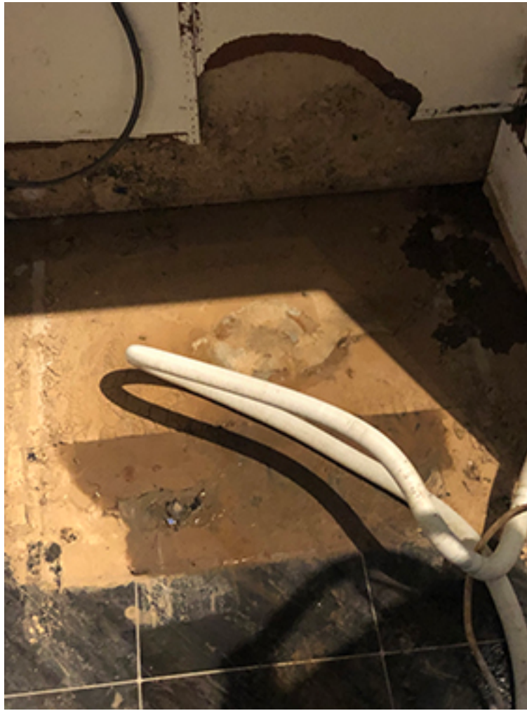
Fig 54/55/6 Kitchen damage behind dishwasher and above kickboard
