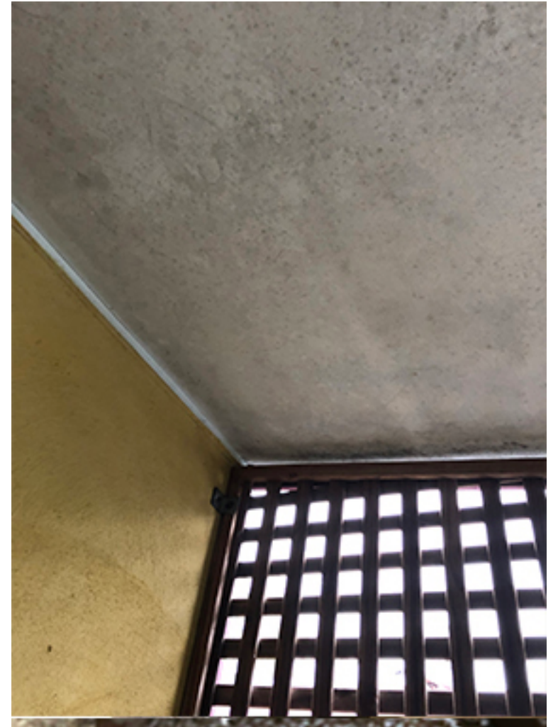
Fig 114/15/16 Mold beginning to show on the eaves - front verandah peeling mold above the door
