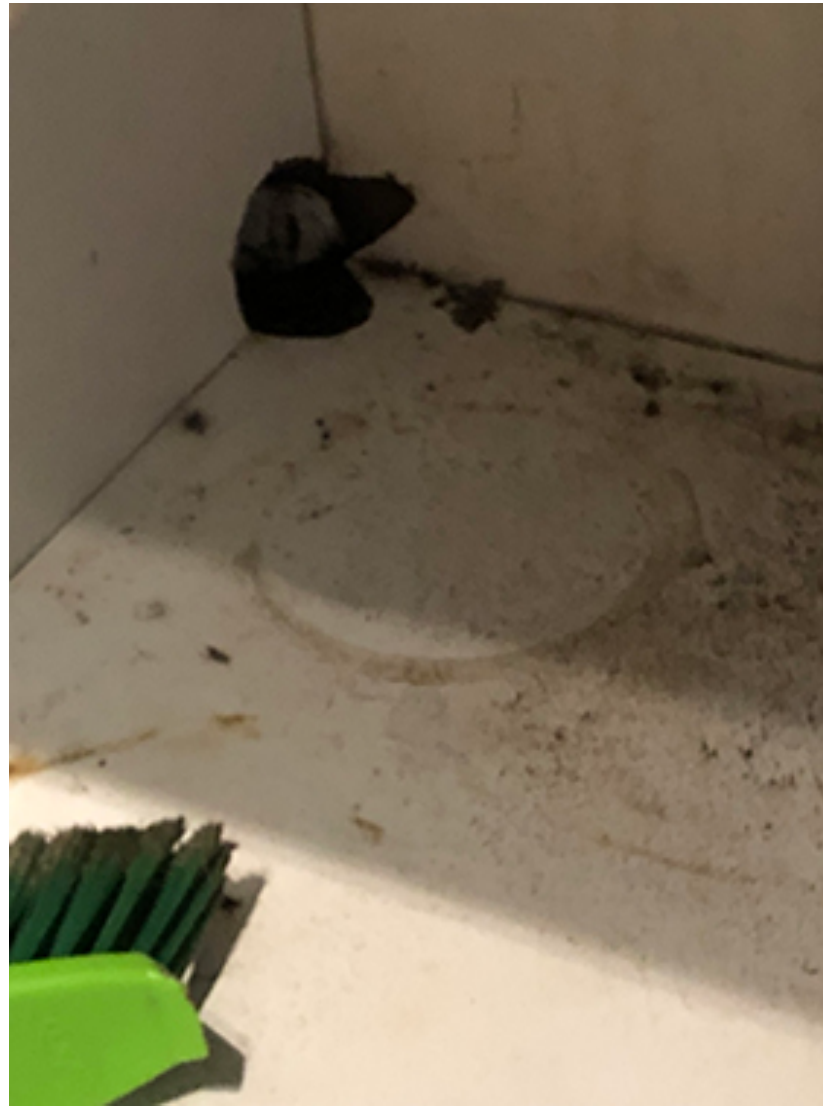
Fig 60/61/62 Kitchen inside cupboards peeling and lifting, stinking inside, everything is effected by the mud dust and mold
