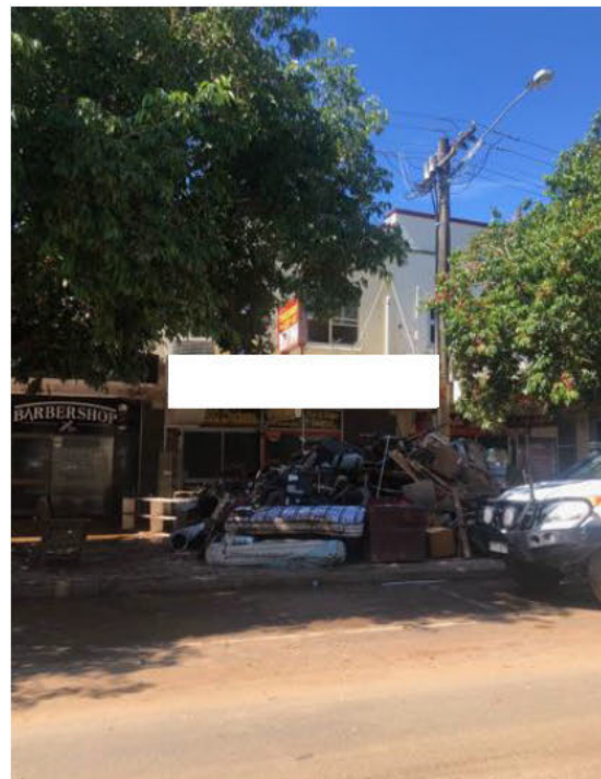
Post FEB 2022 - Commencement of demolition
