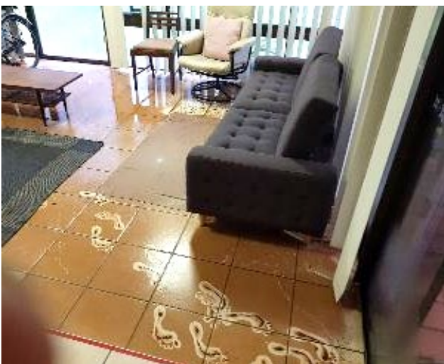
Water nearly gone in sunroom – footmarks in mud
