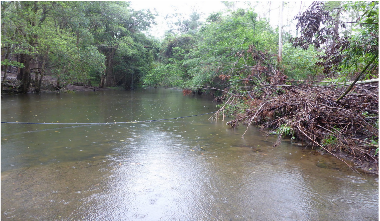
Fig 5: Showing Telstra cable crossing Dingo Creek at Syds Bridge after Bush Fires Jan 2020.
