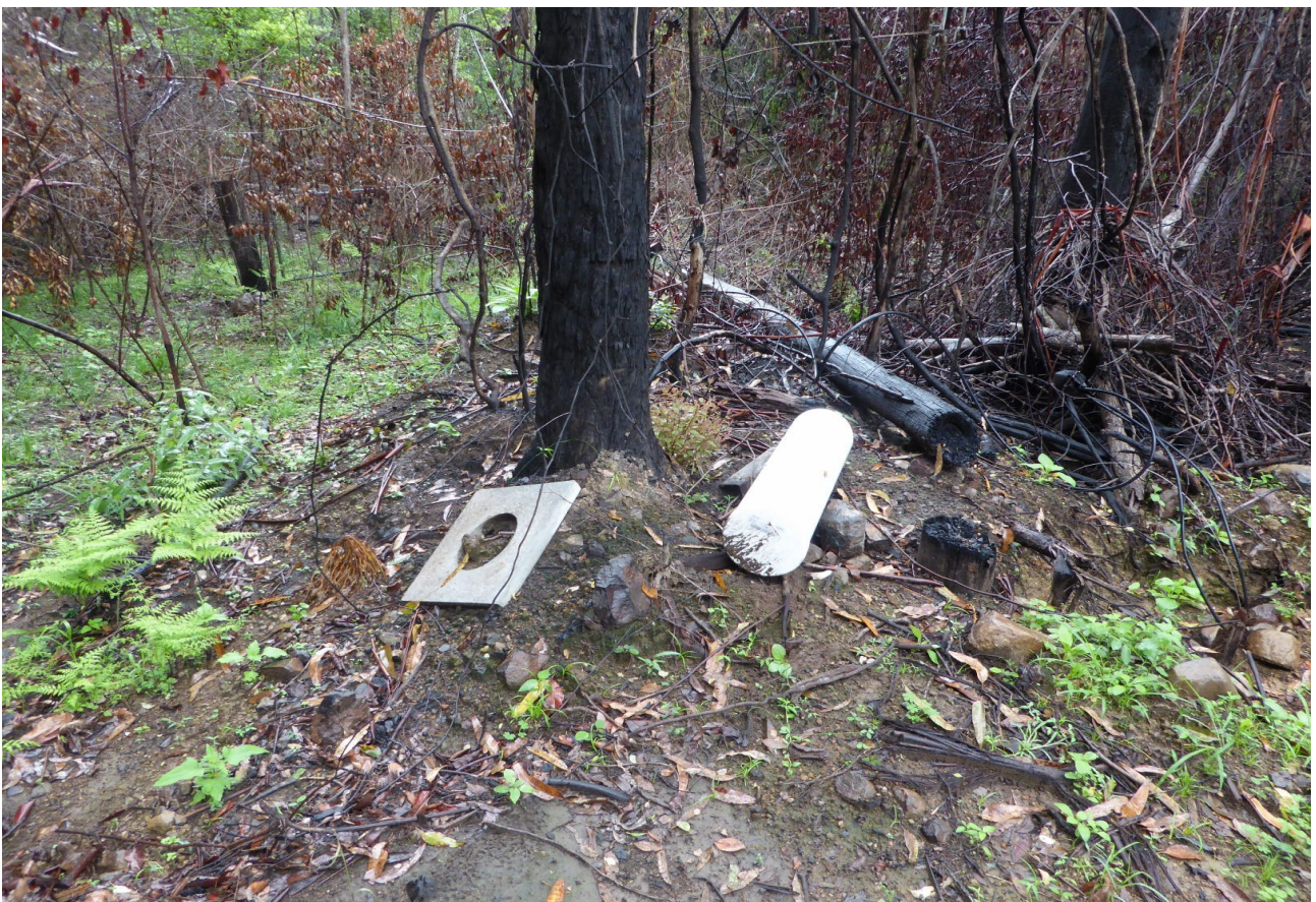
Fig 6: Showing Telstra telephone pole and node after Bush Fires, Jan 2020
