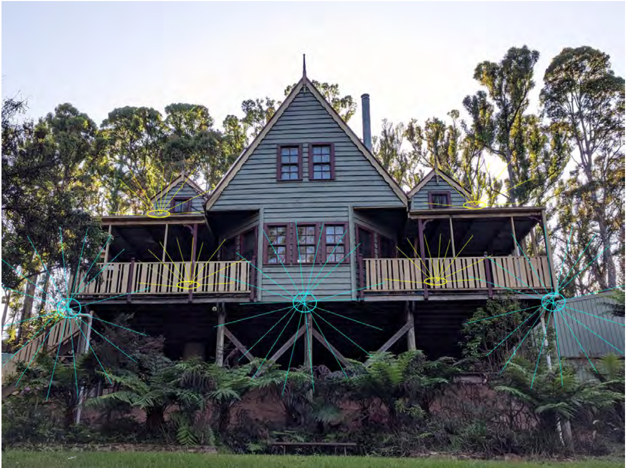
Figure 12: Sprinklers on face of house
