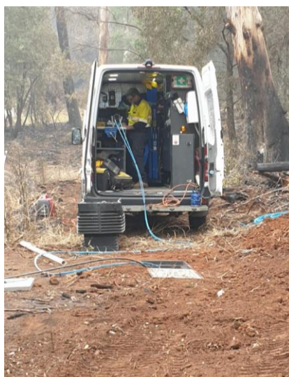
Figure 5: Field technician repairing damaged optic fibre cable, Butchers Ridge VIC
