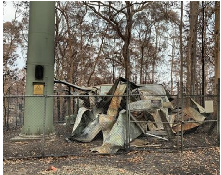
Figure 3: Fire-damaged mobile network facility, Surf Beach NSW
