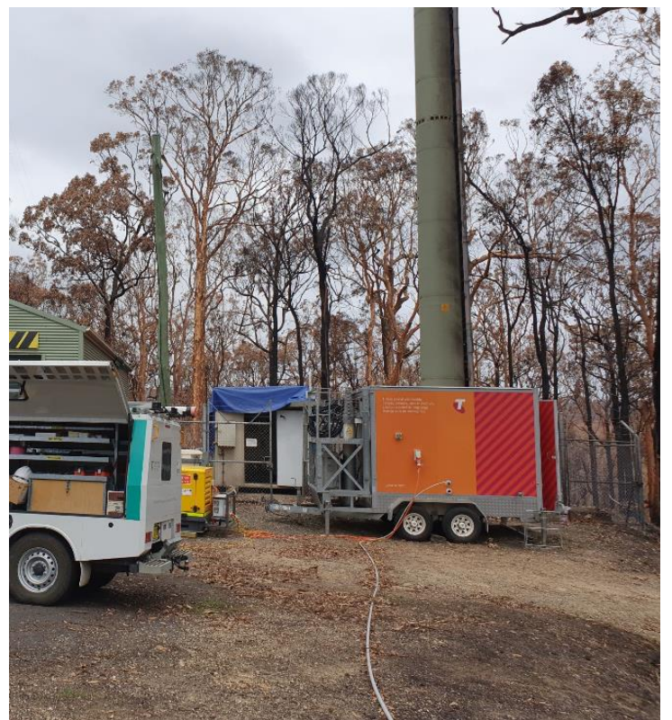
Figure 4: Cell on Wheels with fire damaged mobile network facility in the background (blue tarpaulin covering), Malua Bay NSW
